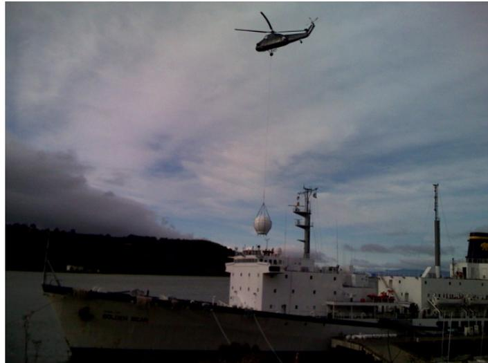
**Satellite Antenna Lowered by Helicopter onto Pedestal**
